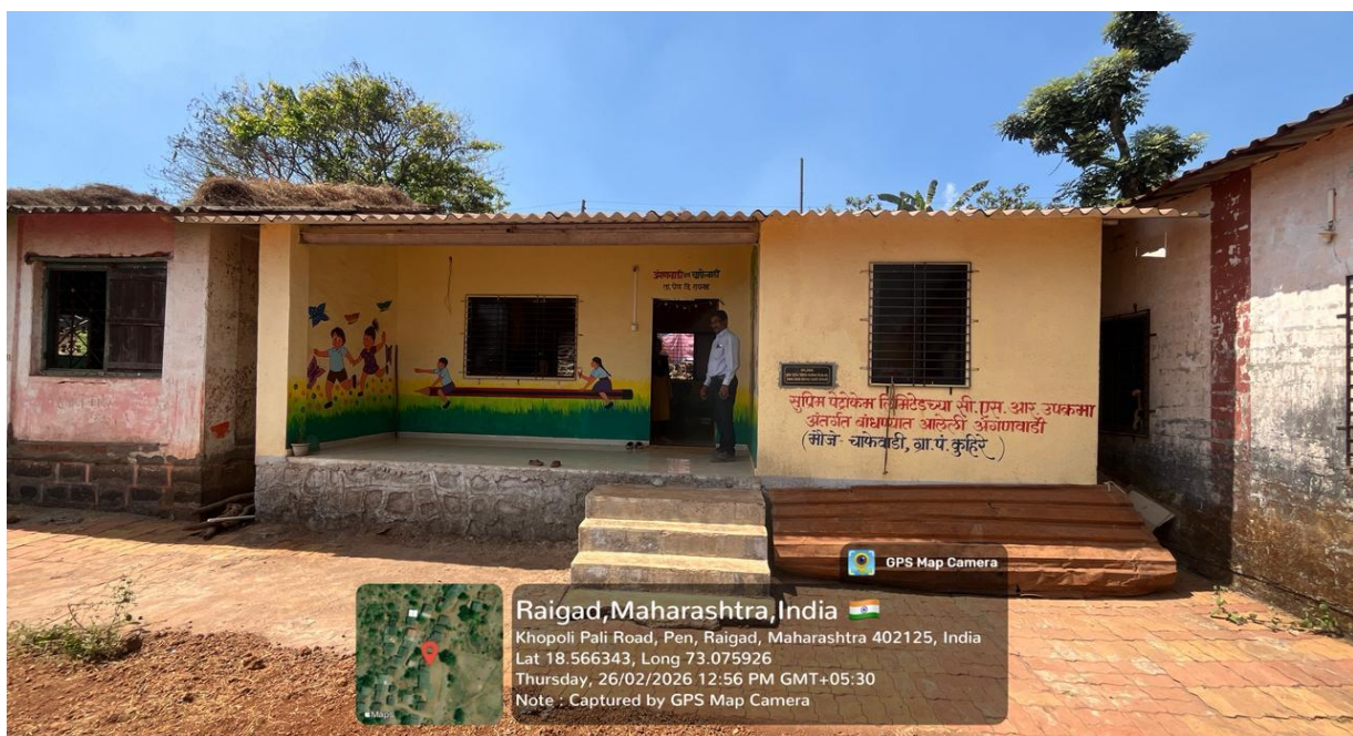
Figure 10: Chafewadi village Anganwadi new building
